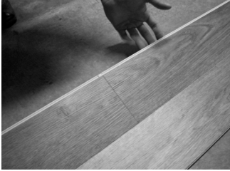
Fig. 6 - Locking long side with ends already locked
