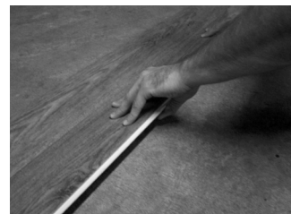
Fig. 4 - Angle long side into prior row.
