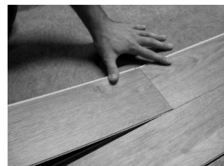
Fig. 5 - Angle end of next plank
